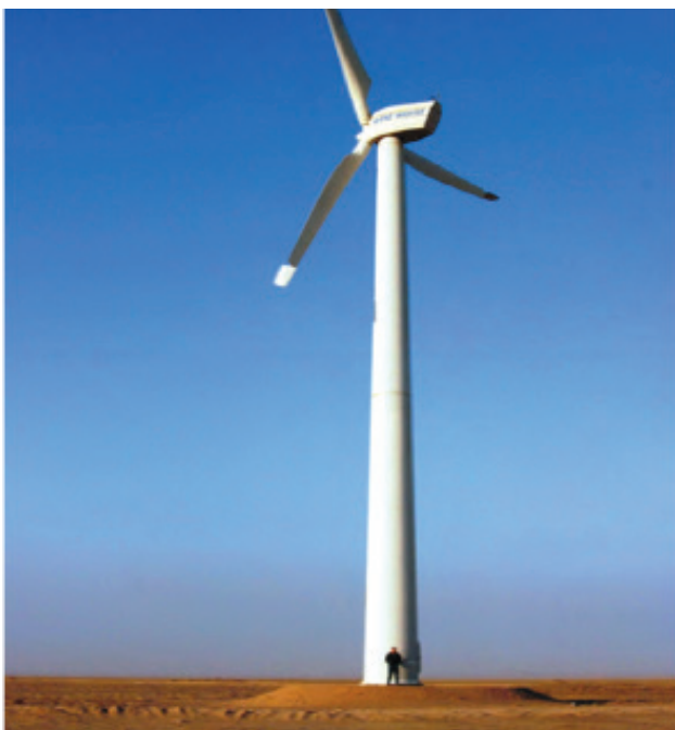
FIGURE 3: 220 kW Wind Energy turbine at Walvis Bay
